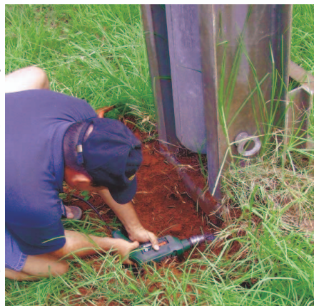
Philip gets down and dirty. Putting an earth on the tower.
